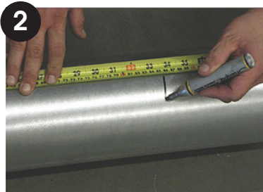
2 Mark standard 5' duct 3 - 4" shorter than length needed.
