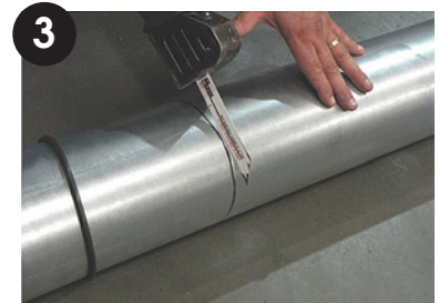
3 Use O-ring (comes with nipple) to mark cut line. Cut.
