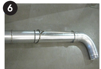
6 Clamp ends of assembly and then clamp O-ring to nipple.
